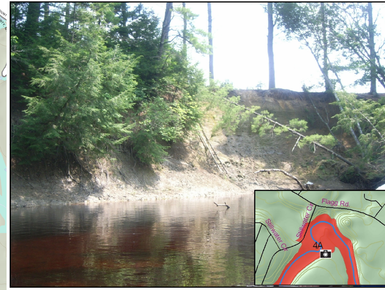
Figure 2: Bank erosion (road bank) and mass wasting in "extreme" sensitivity reach.
