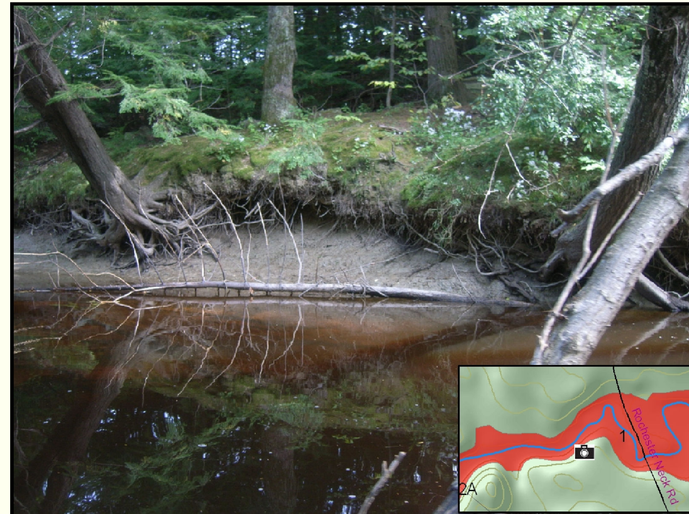
Figure 1: Bank Erosion (right bank) with overhanging trees and exposed roots, in "extreme" sensitivity reach.
