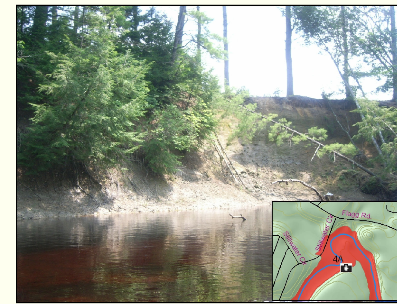
Figure 2: Bank erosion (road bank) and mass wasting in "extreme" sensitivity reach.
